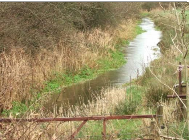
Plate 84: main branch of Aggard flowing from the east (view u/s) (8-1-2012)
