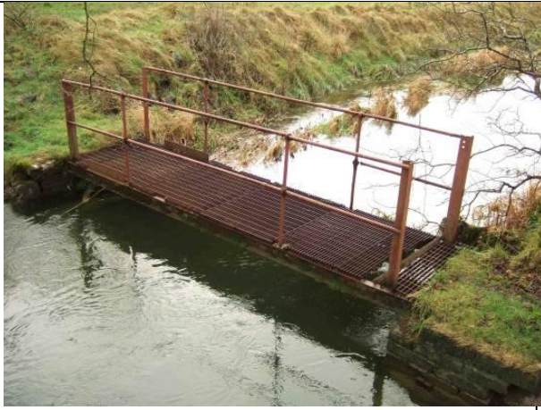
Plate 67: Metal footbridge at AG 10 - view u/s (8-1-2012)
