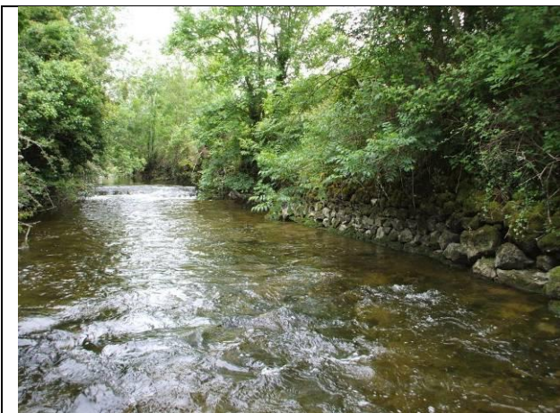
Plate 11: View US from approx. 50m US of Killeely Beg Bridge showing step-run-glide sequence and block armour on left bank (20-7-2011)
