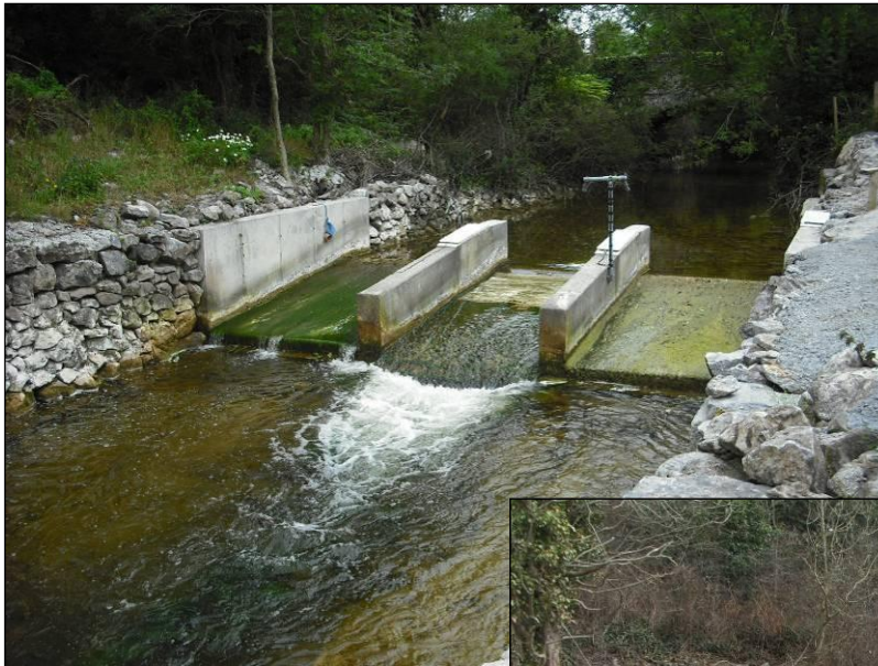
Photographs No. 22 and 23 Existing Salmon Counter
