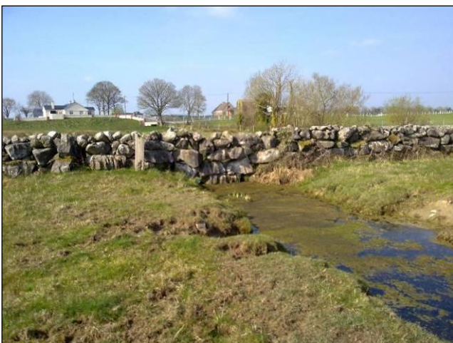
Photograph No. 11 Typical Boundary Crossing along the Aggard Stream in Cregaclare
