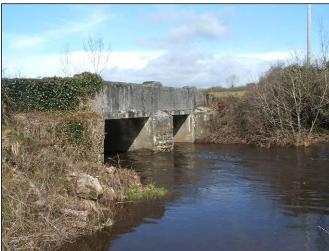
Photograph No. 8 Rinn Bridge taken from the upstream left bank
