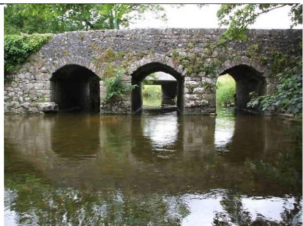
Plate 48: View upstream over shallow glide/run towards old bridge at Craughwell, with the N6 Bridge visible beyond. Crayfish were abundant under boulder/cobble in this stretch.
