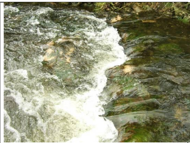
Plate 6: Short step / weir at the head of a run, downstream of the salmon counter at Killeely Beg Bridge (21-7-2011)
