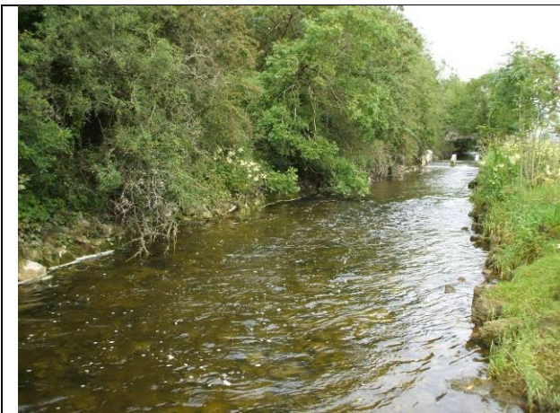
Plate 9: View upstream from approx. 100m D/S Killeely Beg Bridge showing true left bank with extensive rip-rap reinforcement and right bank of rock cut with crevices that would provide good refuges for crayfish (20-7-2011)
